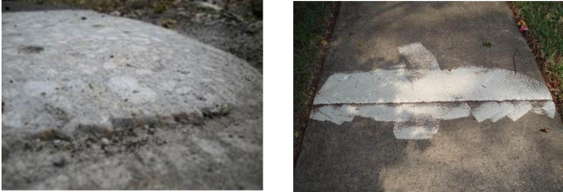
Figure 8: Typical Results from a Grinder
