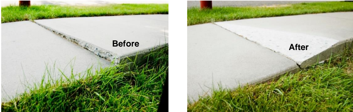
Figure 7: Precision Sidewalk Safety Work Example
